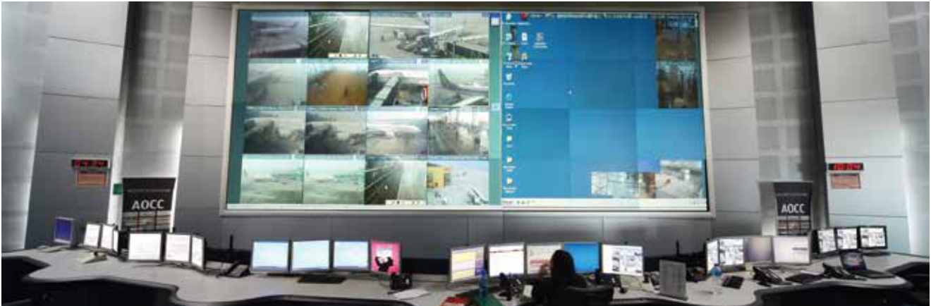
State-of-the-art Airport Operations Control Centre (AOCC) with 4m x 7m Video Wall
